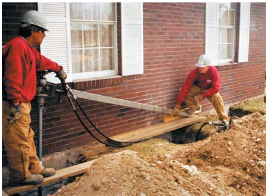
Helical pile installation by hydraulic driver
