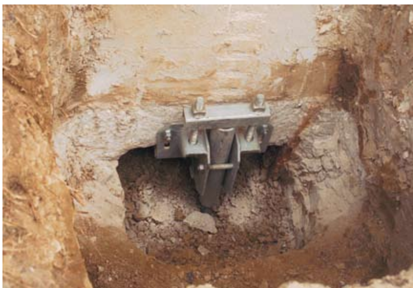
Completed helical pile and bracket
